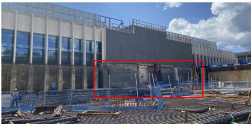
Sample 2 – Building C 1980's Retaining Wall in-situ
