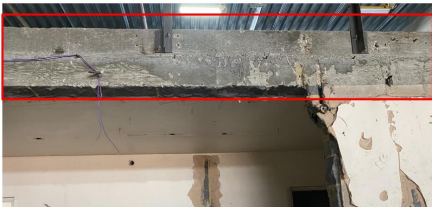
Sample 3 – Building D 1960's Mezzanine Slab in-situ
