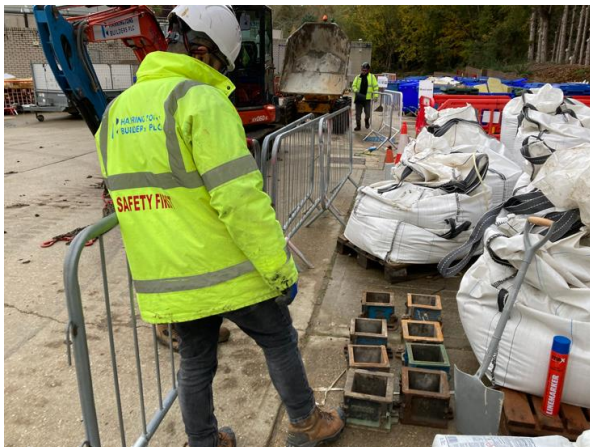
Figure – Cubes for testing being poured on site.
