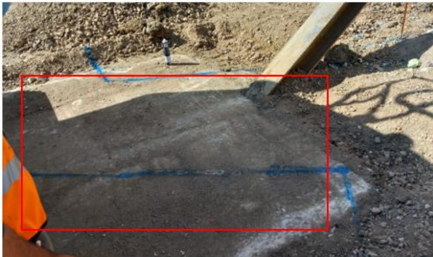
Sample 1 – Building H 2023 Thrust Blocks in-situ
